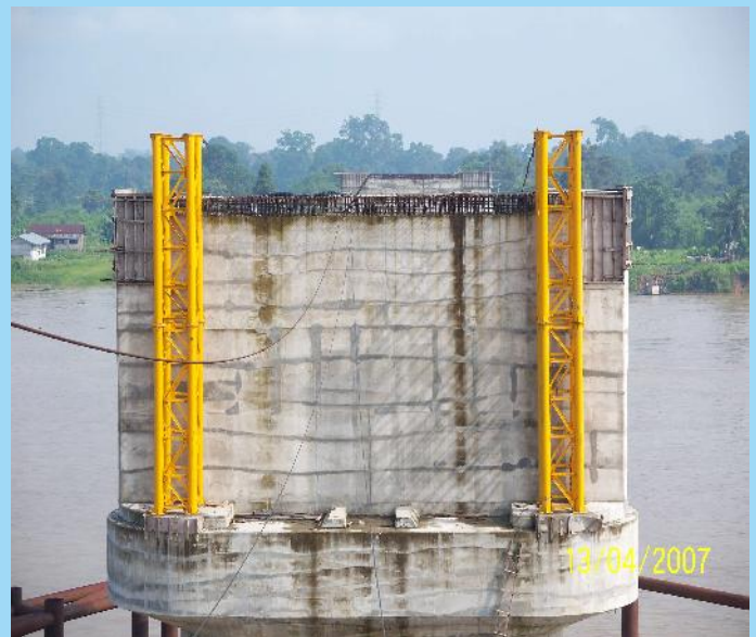
Pemasangan Temporary Tower
