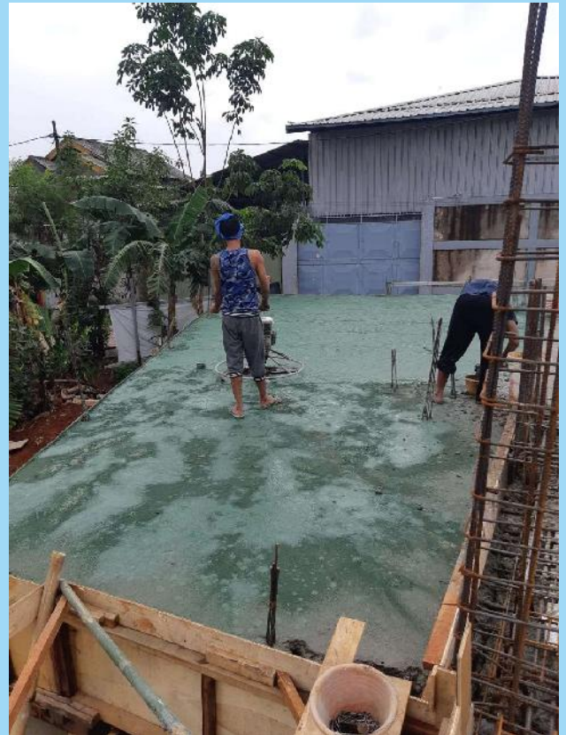
FINISHING FLOOR HARDENER MASJID AL - IKHLAS
