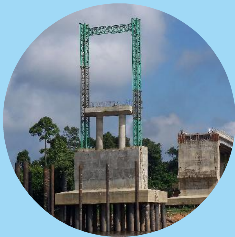
Pemasangan Temporary Tower
